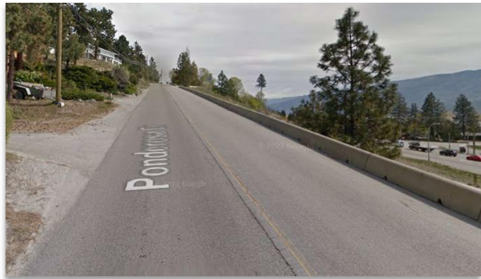
Figure 2-2: Ponderosa Drive Confined Corridor Example (Google Streetview, 2015)
