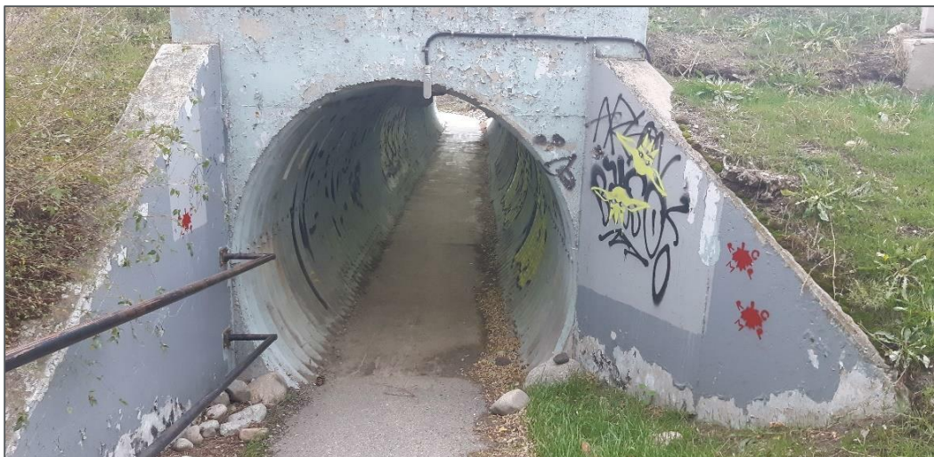
Figure 2.7: Pedestrian Underpass at Princeton Ave Crossing
