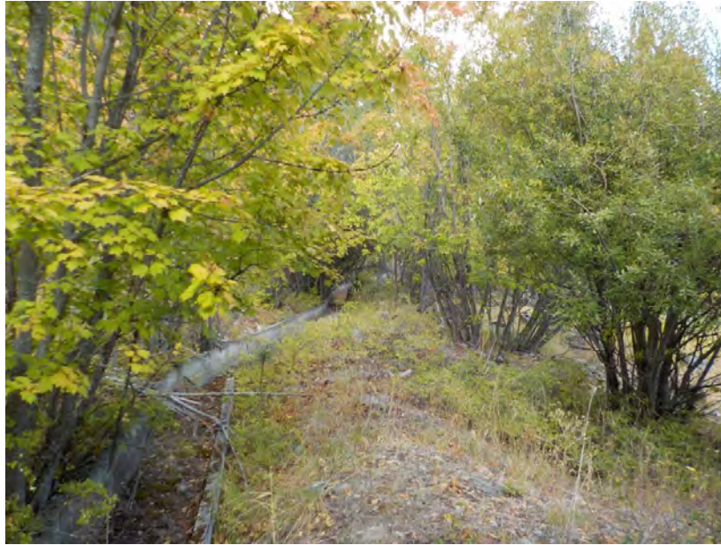
Photo 4. View of a non-functional flume running diagonally through the property from the southwest to northeast corners (August 21, 2018).
