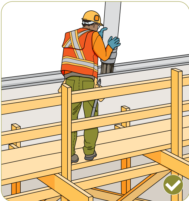
A single-pole wood scaffold can provide a safe work platform for placing concrete.
